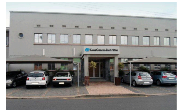
Guala Closures plant in South Africa
